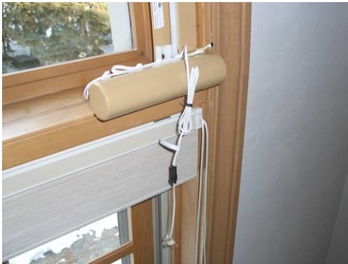
Motor/track assembly shown mounted in window.
