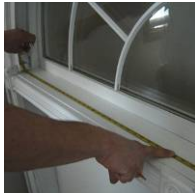
Measure window diameter.
