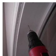
Drill pilot holes.
