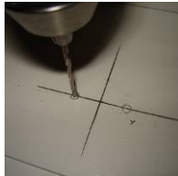
Drill pilot holes.
