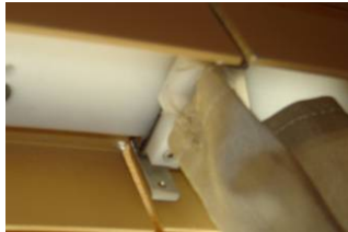
Insert last connector into plastic receiver.
