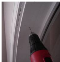
Drill pilot holes.
