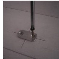
Screw keeper plate to sill.
