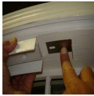
Slide shade stop under track.
