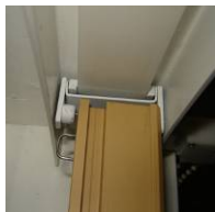
Engage fingers in shade carrier.
