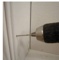
Drill pilot holes.
