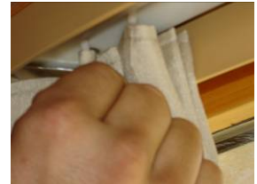
Insert connectors into track.
